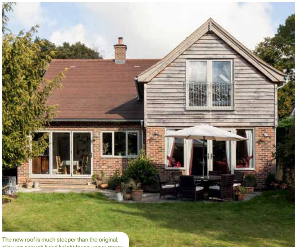
The new roof is much steeper than the original, allowing enough head height for an upper storey
